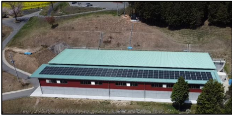
Compost field (solar power generation system)
